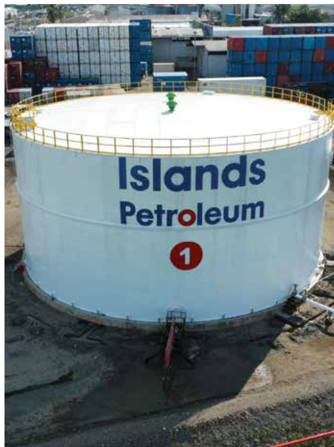
Islands Petroleum's new 5 million litre storage tank in Lae.
